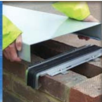
Clickfix coping is produced from aluminium sheet and specially extruded aluminium straps with a neoprene rubber seal. With a unique push & click design it is easy to install and totally weatherproof making it the ideal solution particularly for renovation projects and low-rise buildings.
