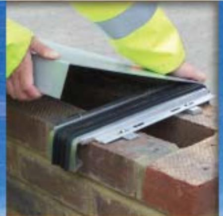
Architectural coping is produced from aluminium sheet and specially extruded aluminium straps with a neoprene rubber seal. A unique rotate & lock design provides weatherproofing and resistance to strong winds making it the first choice solution for high-rise buildings.
